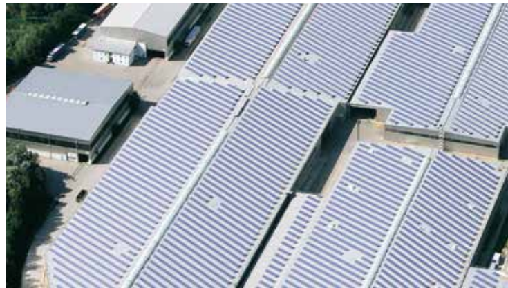
The RIB-ROOF metal roofs for the “Fischer warehouses in Dingolfing, Germany” had been built after one another from 1989 onwards. Photovoltaics were subsequently installed perforation-free in 2005.
