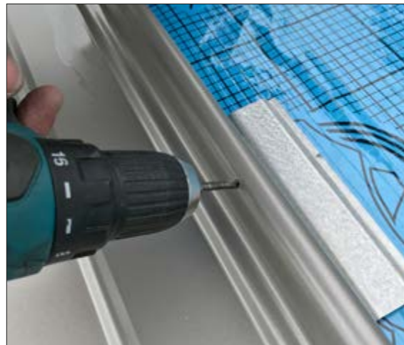
2. Drill a lateral hole on the circular seam at an angle of approx. 45°
