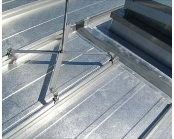
Welded-in dome light with dilatation band; lightning protection bracket
