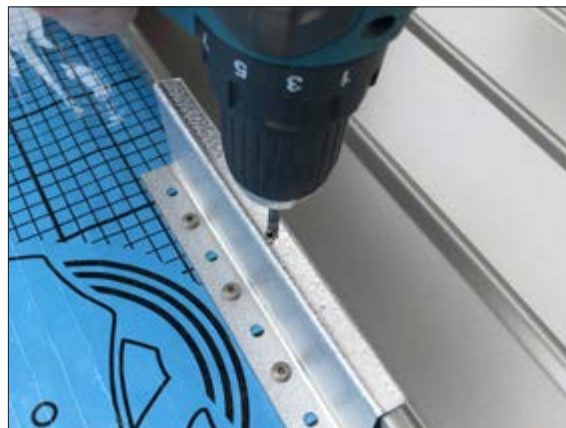
2. Drill a hole perpendicularly at the top of the turned directional clip
