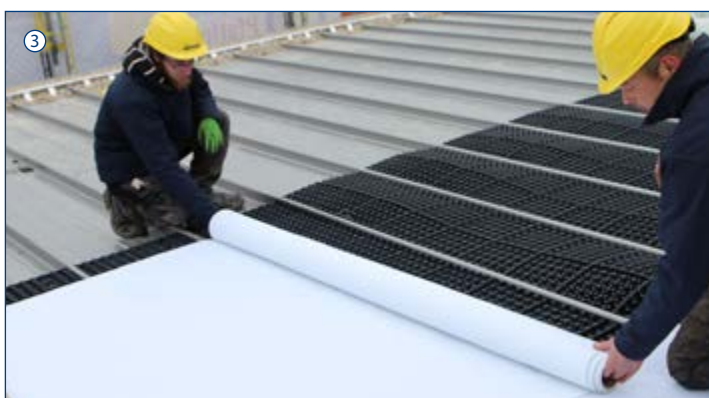
Roll out the filter fleece crosswise to the roof pitch over the drainage and storage layer.
