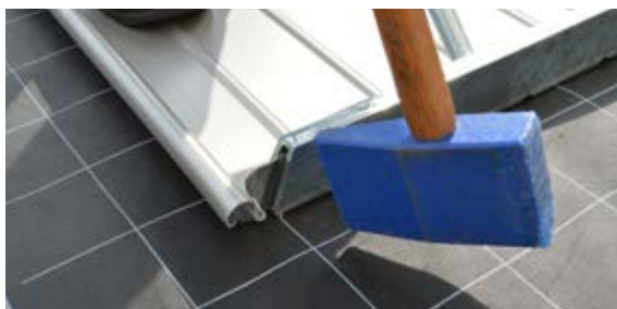
5. Knock with plastic hammer during installation.
