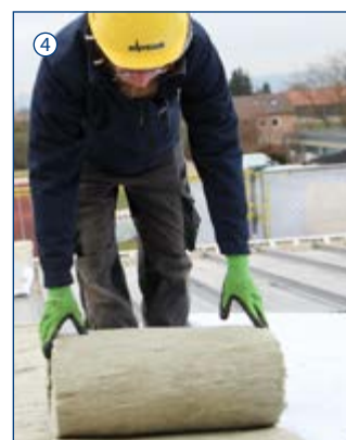
Roll out the Green Roll growing media tightly crosswise to the drainage and storage layer. Leave out the gravel strips or areas. Cut the Green Roll growing media to size if required.
