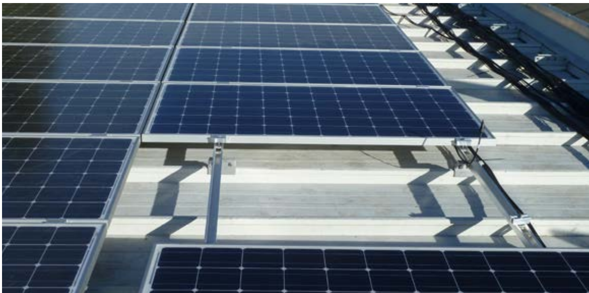
Installation parallel to the roof
