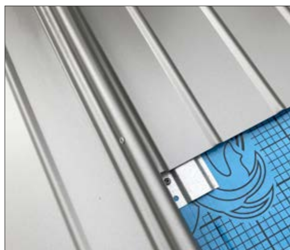
4. Finally, swivel in the next profiled sheet
