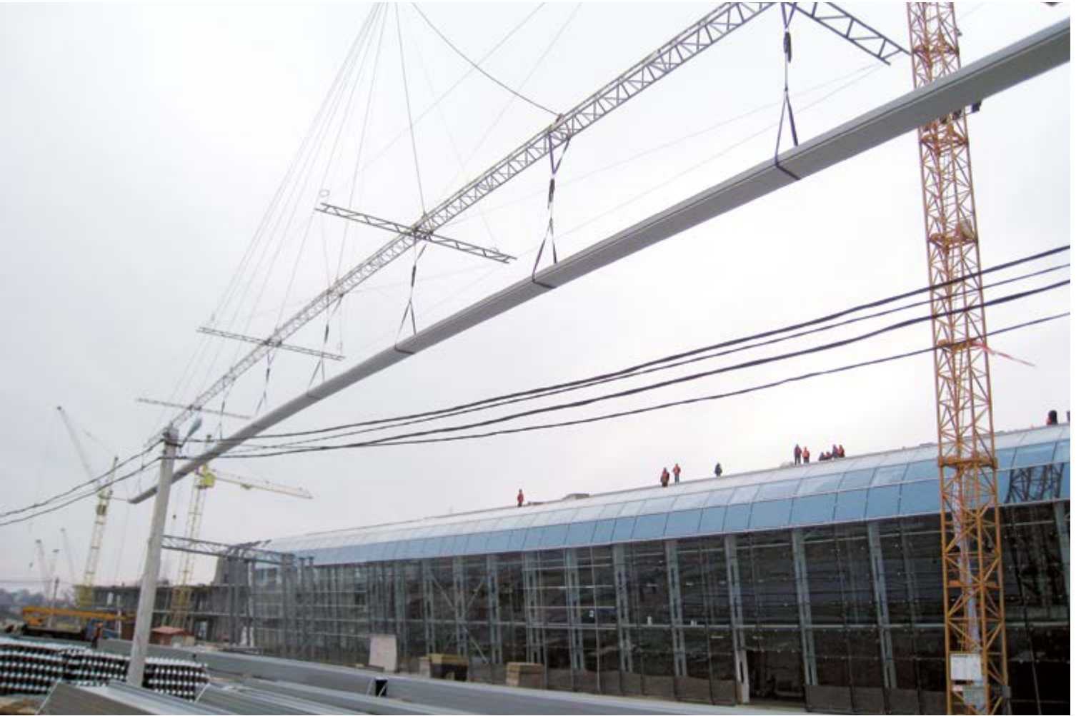
Special spreader beam for extra long profiled sheets.
