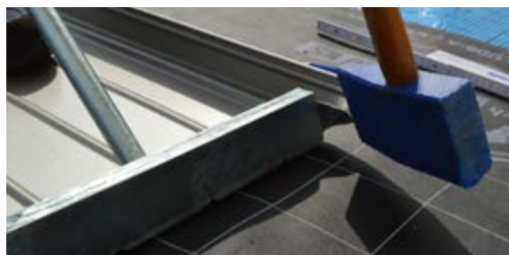
6. Set up bottom boom up to 90° and then check.
