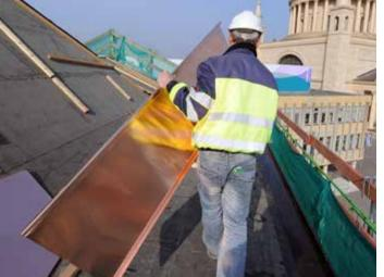
For the implementation of simple roof surfaces, manual produced metal roofs often get carried out with an angular standing seam. The non-self-supporting sheets are usually applied to full-surface substructures and fastened indirectly with adhesives. For larger lengths, transversal joints must be formed. The angular standing seam roofs are made of the materials copper, titanium zinc, aluminum and (stainless) steel.
