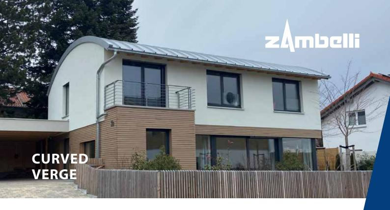
A roof termination that is made to be seen! Especially for smaller roof radii and buildings with special visual requirements, Zambelli offers a particularly appealing variant. Instead of a polygonal design with short lengths, individual rounded segments of the verge termination correspond precisely to the radius of the roof construction.
