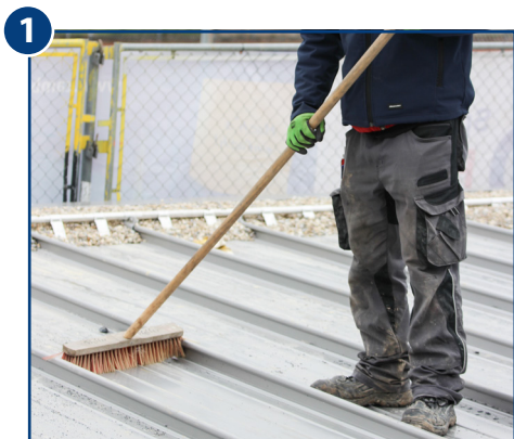
Sweep the RIB-ROOF profiled sheets.
