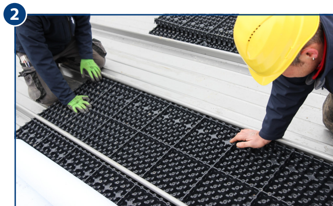
Install the drainage and storage layer tightly butted without overlapping and with the holes facing upwards. Ensure that the edges of the drainage and storage layer are positioned under the RIB-ROOF profiled sheet seams.
