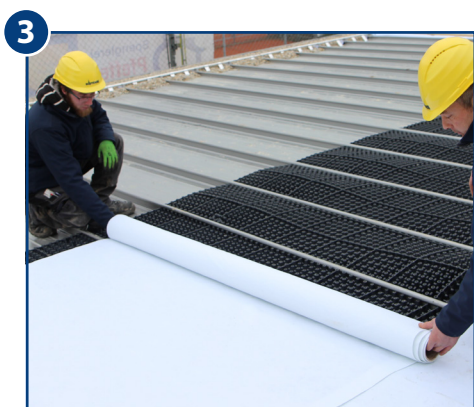
Roll out the filter fleece crosswise to the roof pitch over the drainage and storage layer.
