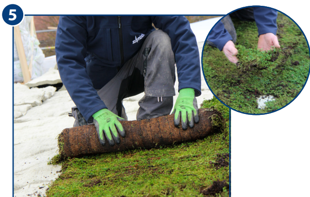
First align the Sedum Mix vegetation layer, then roll it out carefully and tightly crosswise to the Green Roll growing media. If necessary, cut the Sedum Mix vegetation layer to size using scissors or a utility knife with a hooked blade. Ensure that the Sedum Mix vegetation layer covers the entire Green Roll growing media.
