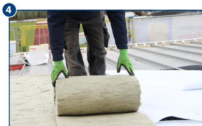
Roll out the Green Roll growing media tightly crosswise to the drainage and storage layer. Leave out the gravel strips or areas. Cut the Green Roll growing media to size if required. Thoroughly water the Green Roll growing media. Apply Urbanscape slow-release fertiliser evenly on the surface (approx. 30 - 35 g/m²).
