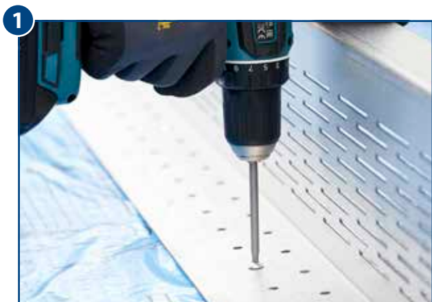
1 Fasten the Thermo-Z spacer profile offset to the top boom of the trapezoidal sheet, or alternatively with equal distances to another substructure.
