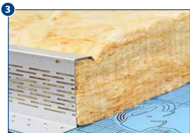
3 When laying the thermal insulation, ensure that the joints fit tightly. In case of installation without high diffusion protective sheet (optional), ensure there is sufficient compression of approx. 20-40 mm.
