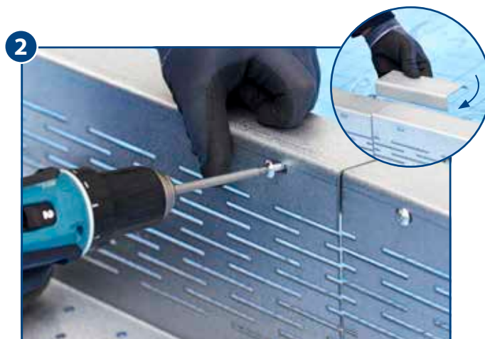
2 Fix the joint connector to both sides of the Thermo-Z spacer profile. Ensure there is an expansion joint of approx. 3-5 mm.
