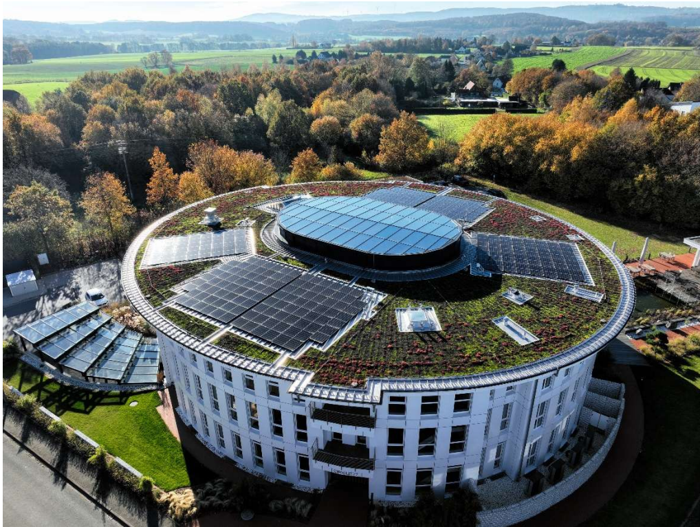
Green roof meets metal roof: A large section of the roof at CIRCLE77 was extensively greened by Zambelli and external partners. The basis for this is the underlying Zambelli metal roofing system. It serves as the load-bearing structure, root-resistant waterproofing layer, and water-bearing level. Photo: Zambelli Holding GmbH.
